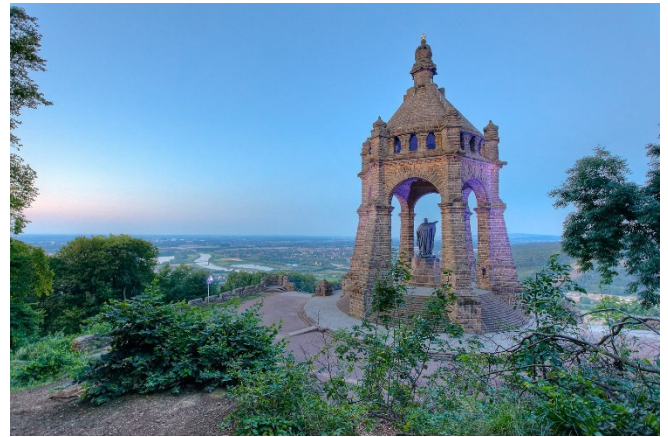
Porta Westfalica CCBYSA Csassenberg-at-wikimedia.commons
