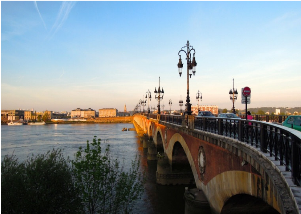
Pont de Pierre, Bordeaux, Aquitaine CCBY David McKelvey-at-flickr
